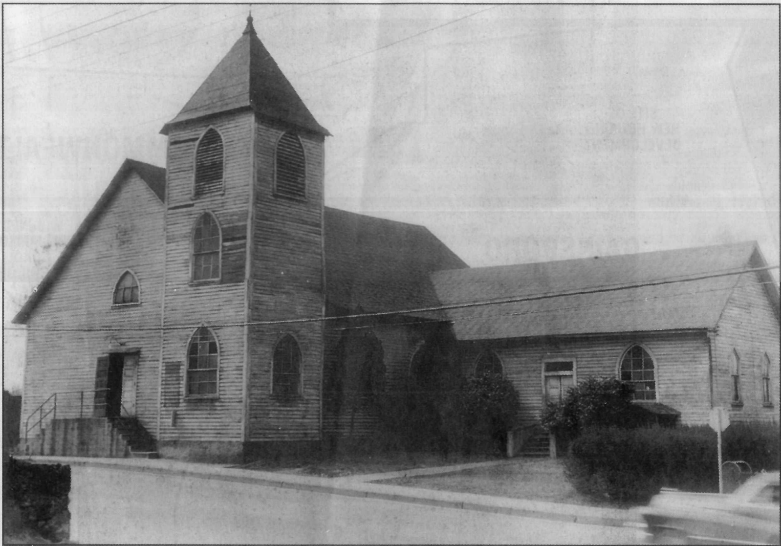
Mount Zion Baptist Church, formed in 1884, has had four buildings. The one at left was its second, built in Northeast in 1908. Mount Zion built its first brick building, renamed Greater Mount Zion, in 1955. It was torn down 15 years later to build the Roanoke Civic Center. The fourth building is on Grayson Avenue Northwest.
